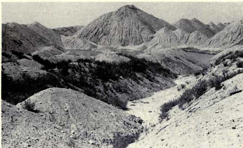
Draglines often deposit the material in conical piles or sharply serrated ridges that are steep and subject to severe erosion. (Fig. 6)
