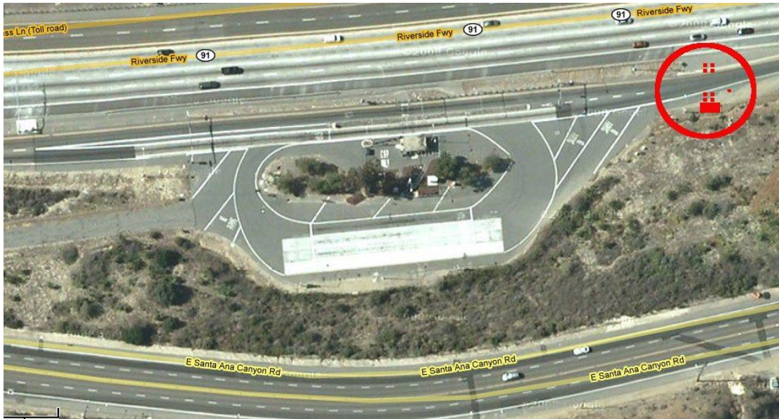
Figure 2. A satellite photo of the Peralta weigh station located on the Riverside Freeway (State Route 91). The scales are located on the inside lane next to the building in the top center and the outside lane is for unloaded trucks. The measurement location is circled at the upper right with approximate locations of the scaffolding, support vehicle and camera.
