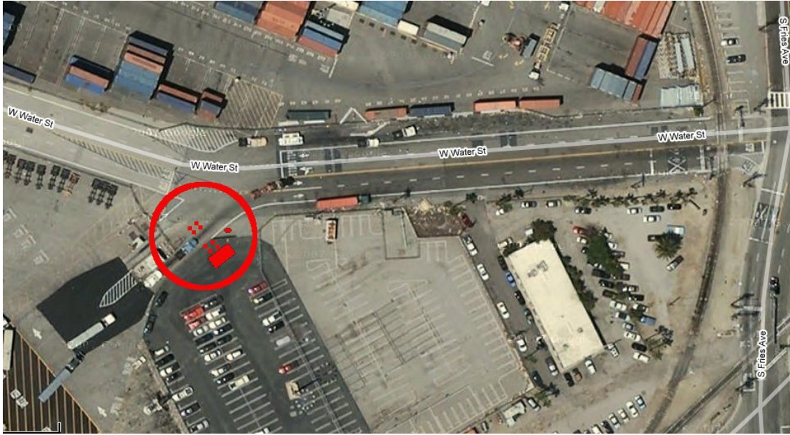
Figure 4. A satellite photo of the Port of Los Angeles Water Street. exit. The measurement location is circled in the lower left with approximate locations of the scaffolding, support vehicle and camera.
