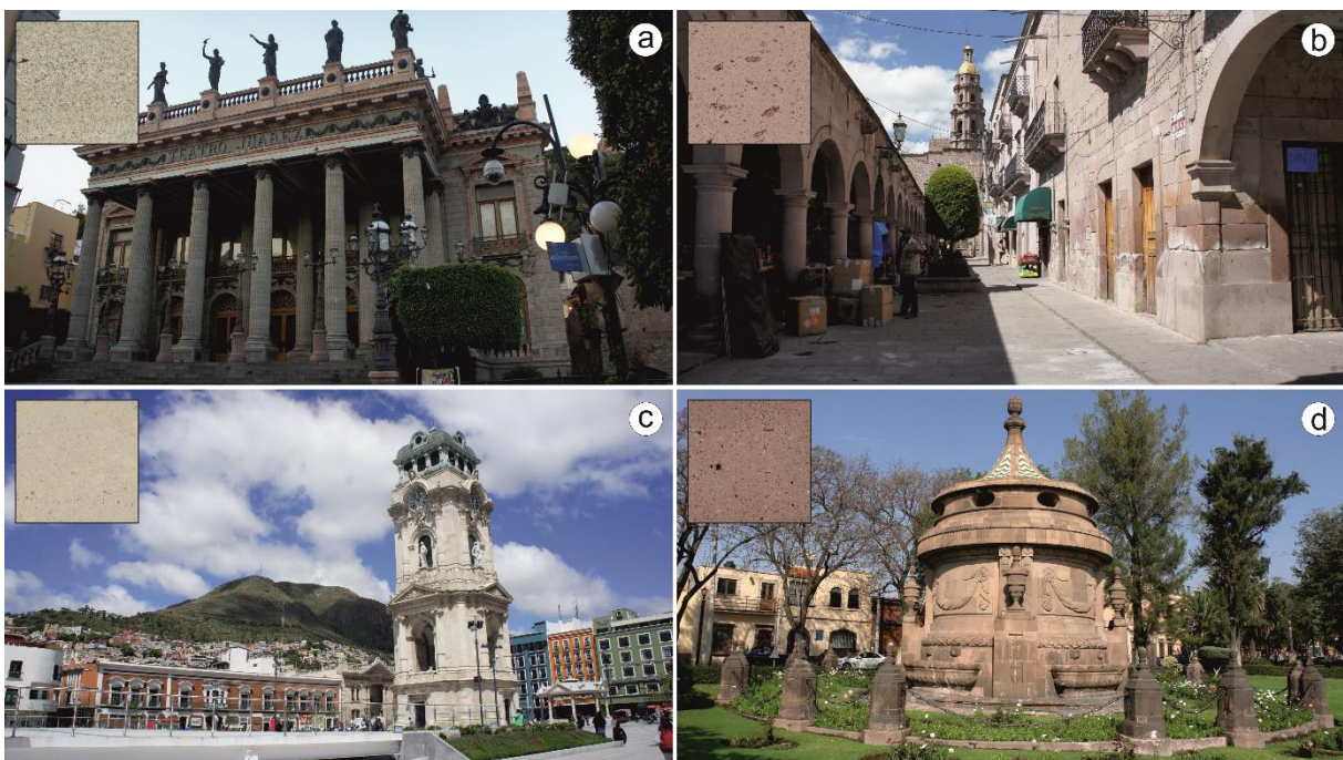
Figure 1.1: Intensive utilization of volcanic tuff rocks in the historic city centers of Central and Western Mexico. a Teatro Juárez in Guanajuato (Loseros tuff). b Marketplace and Parroquia San Miguel Arcángel in San Miguel el Alto (San Miguel el Alto tuff). c El Reloj Monumental de Pachuca in Pachuca de Soto (Blanca de Pachuca). d Caja de Agua in San Luis Potosi (Cantera Rosa).
