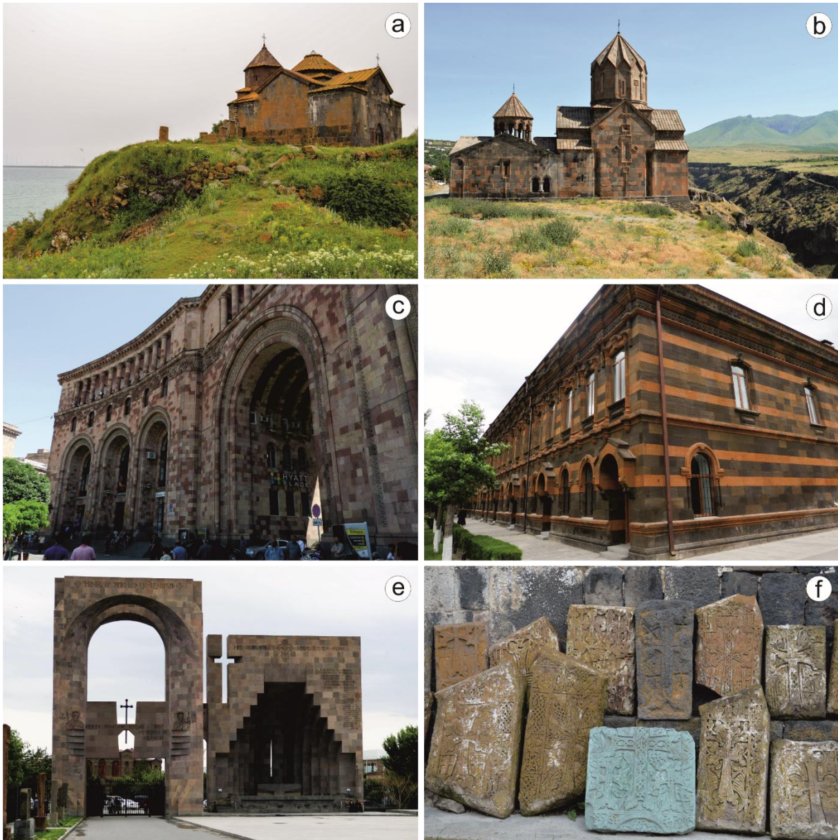
Figure 4.1: Historic buildings and artwork erected with local tuff stones all over Armenia. a Hayravank monastery at the western shores of Lake Sevan. b Hovhannavank monastery at the edge of the Kasagh River canyon. c Characteristic tessellated tuff facade at the Republic Square in Yerevan. d Colorful tuff facade at the Christian Education Center of the Apostolic Church in Etchmiadzin. e Open Air Altar at the residence of the Catholicos in Etchmiadzin. f Khachkars along the gavit of the Sevanavank monastery
