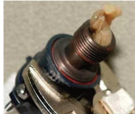
Fig. 2. Biofilm formation inside the condensate plumbing at the inlet to the Russian condensate processor. Image: NASA.
