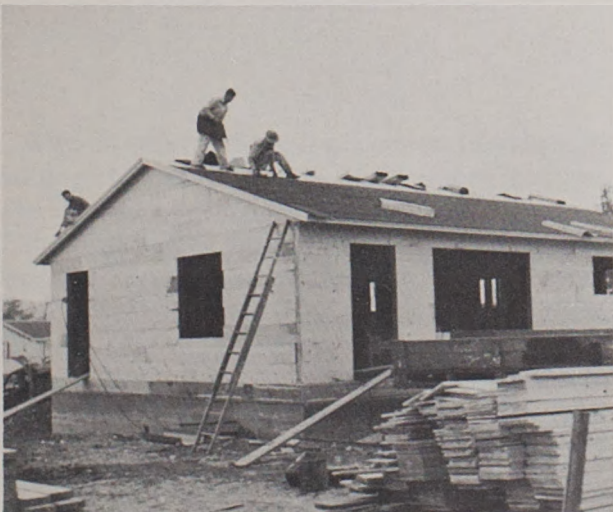
e. Construction of dwellings. . .
