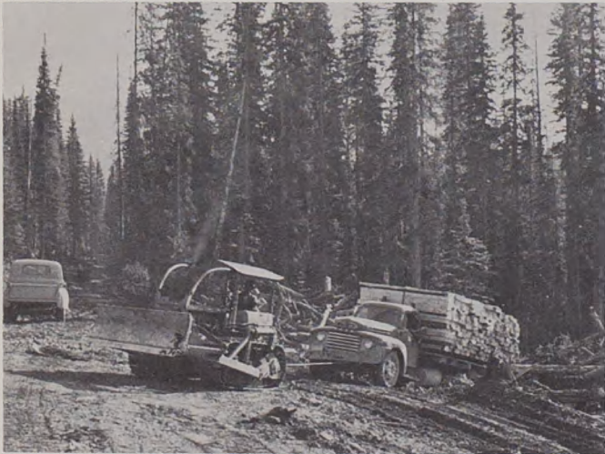
b. Access roads built for salvage. . .
