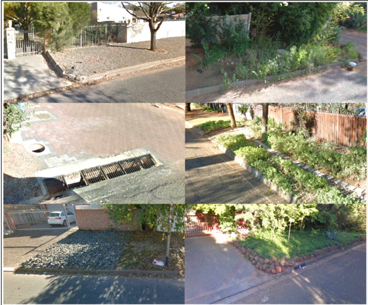
Figure 3.19 Examples of verges and sidewalks that are unsuitable for walking, in Universitas, Bloemfontein City (Source: Author).
