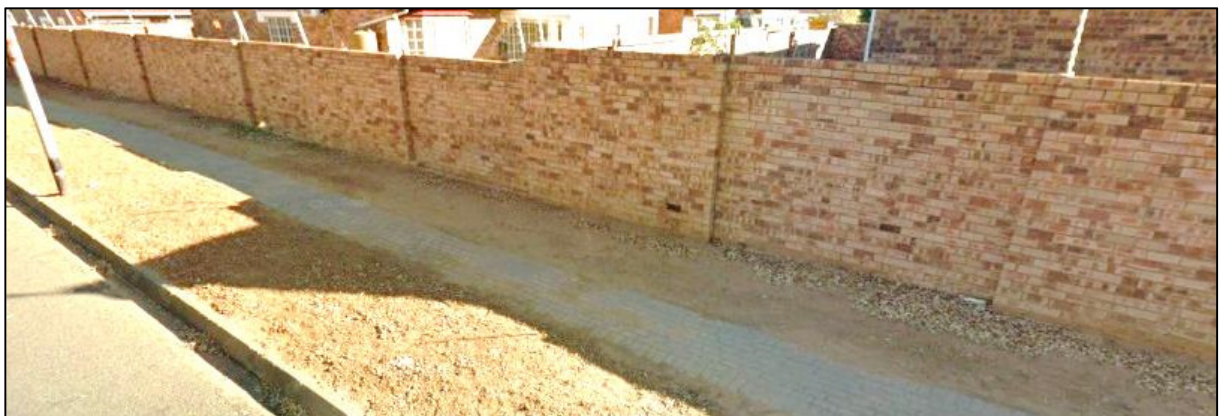
Figure 4.11 Sidewalk location 10; 7 Weitz Street, Universitas (Source: Author).
