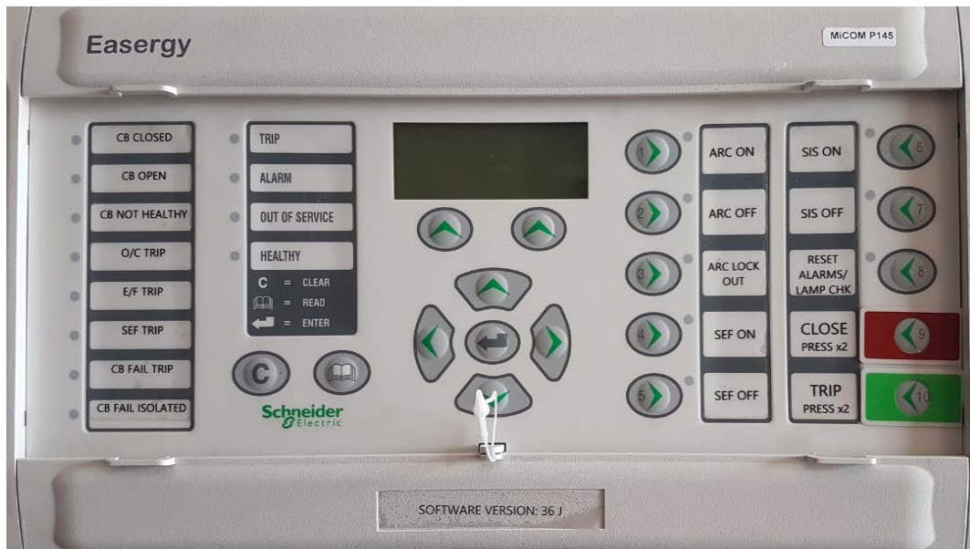
Figure 3.11: MiCOM P145 relay
