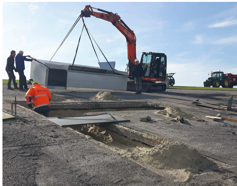
Figure 3: Excavation of the dike slope and placement of the overtopping tanks inside the dike.
