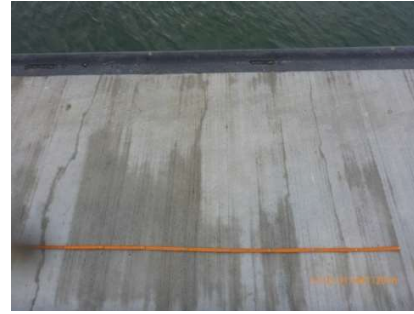
Figure 1: Transverse cracks running across the entire width of the top surface of a newly constructed quay; general view (left); typical crack spacing between 30 and 60 cm (right)
