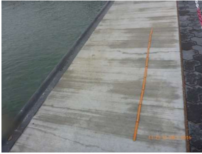
Figure 1: Transverse cracks running across the entire width of the top surface of a newly constructed quay; general view (left); typical crack spacing between 30 and 60 cm (right)
