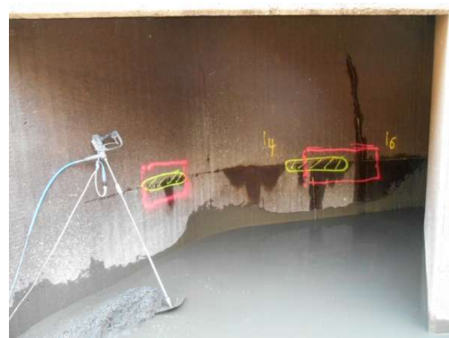
Figure 11: View of the lock, bottom gate, drainage area (left); horizontal construction joint and vertical crack prior to exposure of rebars (right)
