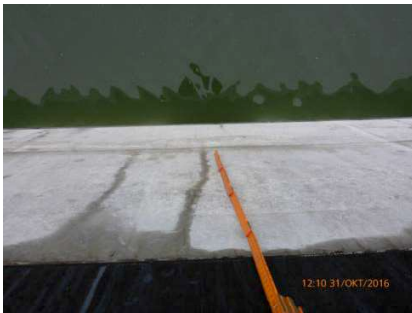
Figure 2: Cracking pattern on the face of the quay (left); cross-section of the quay superstructure (right)
