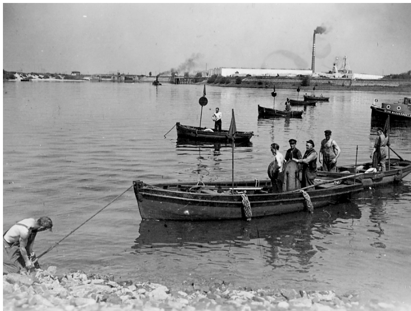
Fig. 8: Plumbing a cross section on the Suederelbe in 1950
