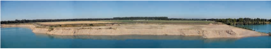
Fig. 3: Steep embankment being dredged against
