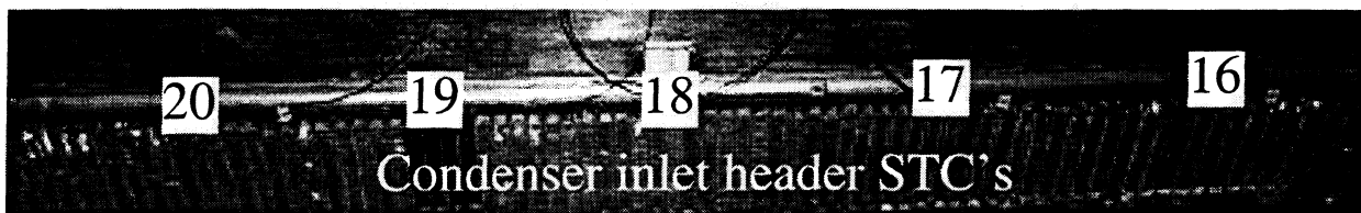
Figure B.9 Condenser inlet header surface thermocouples
