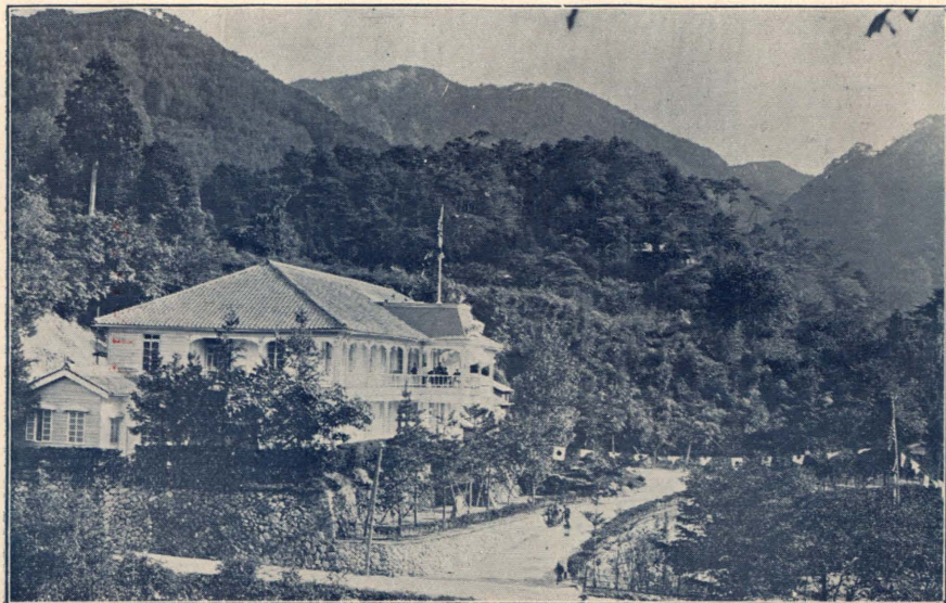
GENERAL VIEW OF THE ARIMA HOTEL.
