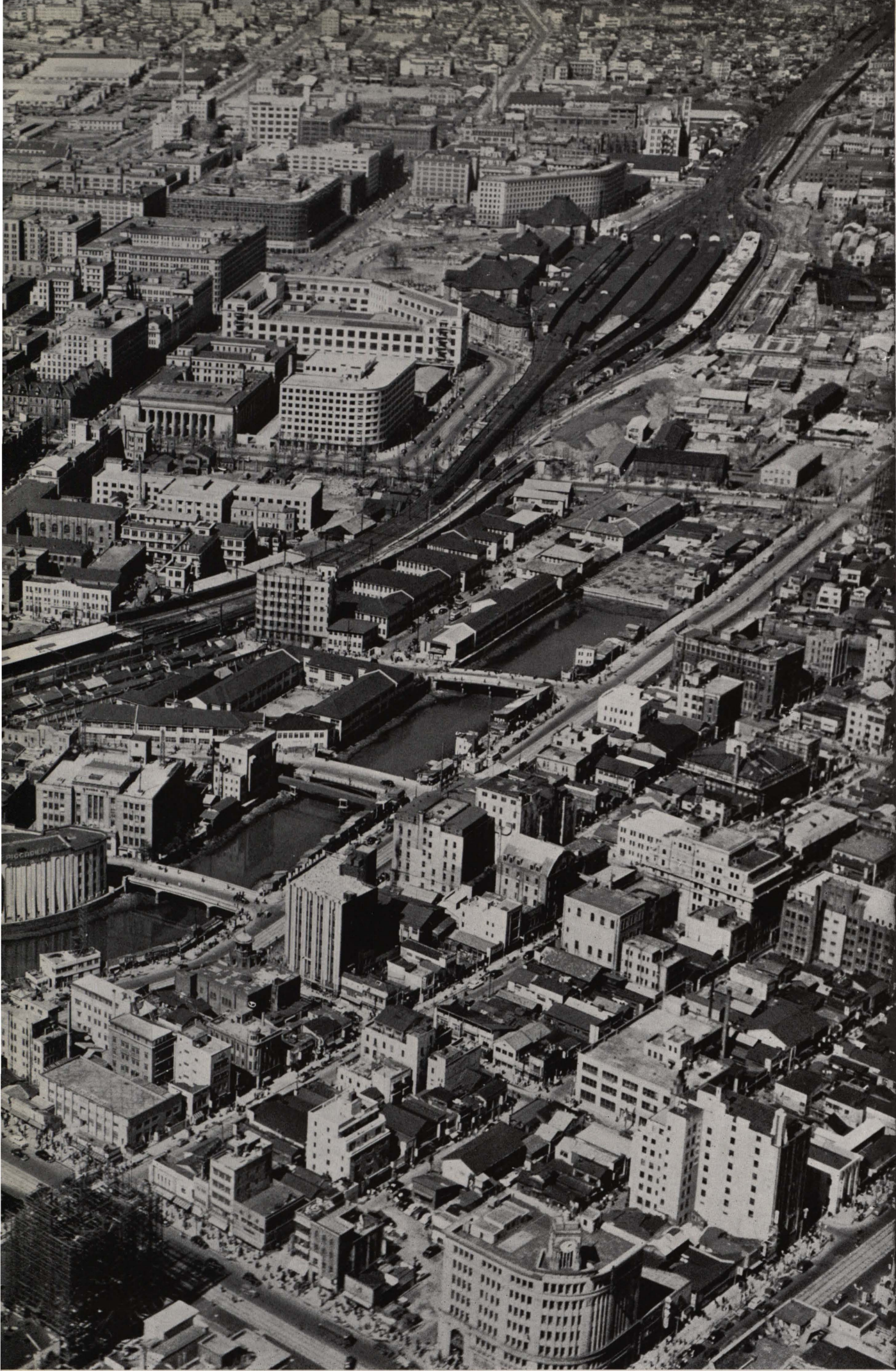
Tokyo, with its population of seven million people, is still changing in appearance. Here is the center of the metropolis with its imposing buildings and wide roads.
