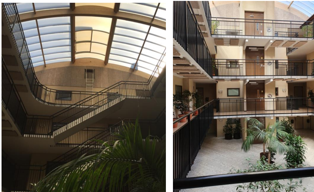
Figure 4.16. The transparent roof with openable hatches over the courtyard at Musteriet (left) and acoustic sound panels under the access balconies (right).
