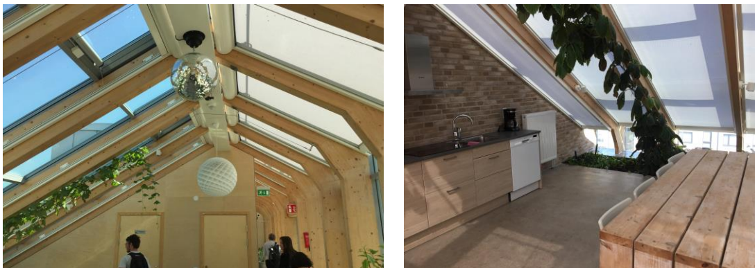
Figure 4.5. The glazed rooftop is divided so that there can be different activities simultaneously, for example parties and meetings.
