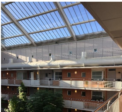
Figure 5.2. Warm air can be blown toward the glass ceiling in wintertime to prevent condensation (Höstvetet).
