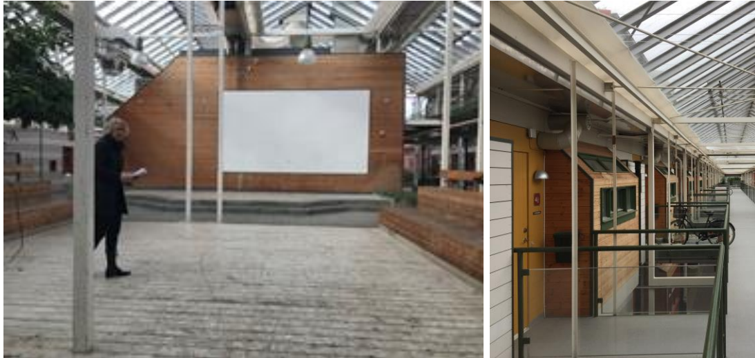
Figure 4.9. The open stage area on the first storey and the (right) openings in the access balcony floors that let more daylight into the first storey.
