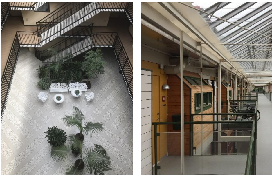
Figure 5.1. Solid access balconies create darker areas (left) while cut outs provide more light (right).
