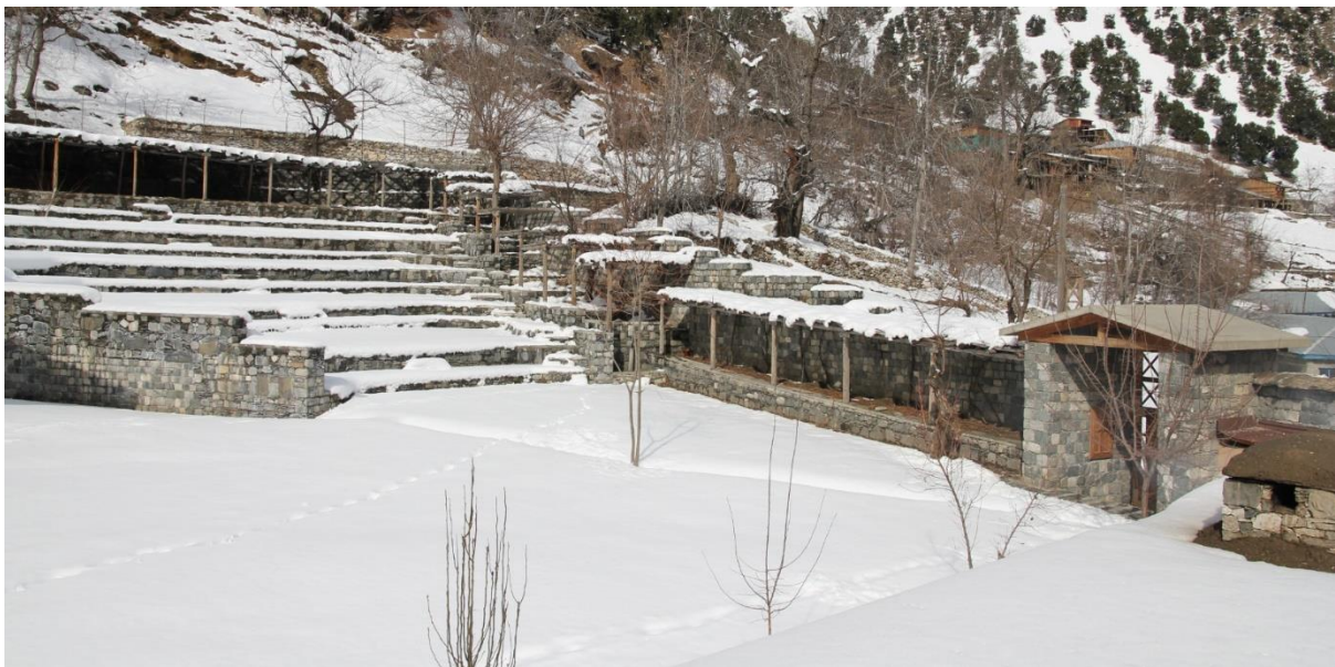
Main building elevation and amphitheatre to the right of the main building.
