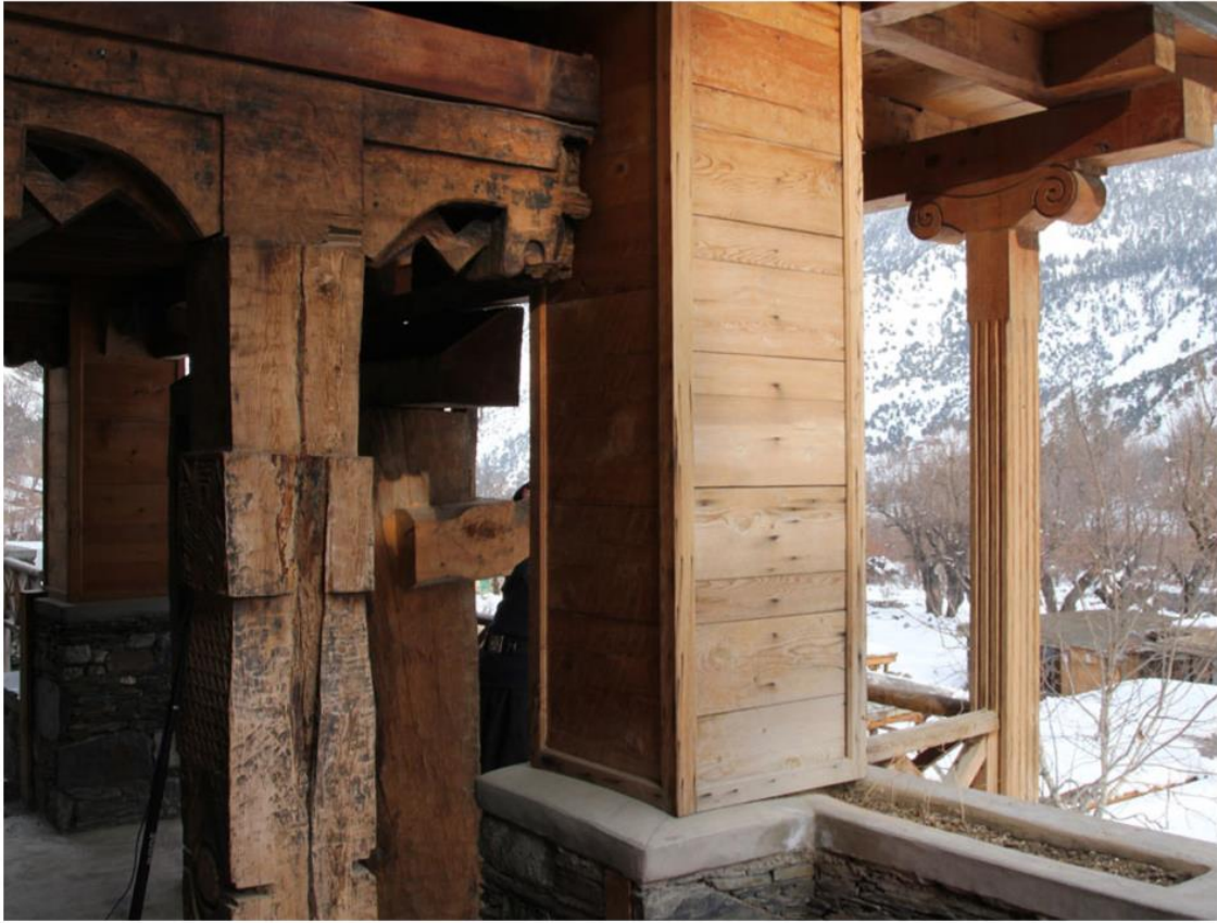
Pillars from removed from Kraka' Jestakhan and built in to the Kalasha Dur, juxtaposed with a version of an ionic column displaying a voluted capital and fluted shaft.
