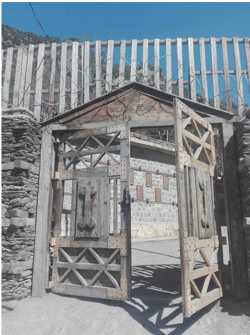
Figure 3.3. The Entrance to Kraka' Kalasha School, built by the Greek Volunteers in the mid 1990s. A Vergina Sun has pride of place, just below the apex of the pediment. (Photograph the author).
