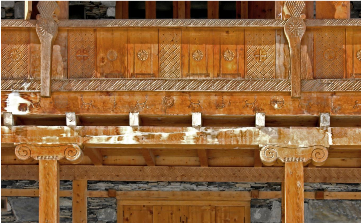
Detail of the façade above the museum entrance. Note the ionic volutes and ovolo on the column capitals. Note also how Vergina suns replace the traditional roundels on the cot'ala thũ' plank columns (see examples in Kalasha houses below). The other motifs are local.
