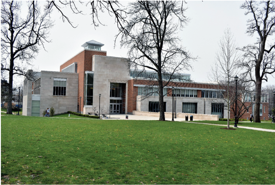
FIGURE 2A. Exterior of the renovated and expanded Gatton College of Business and Economics at the University of Kentucky.
