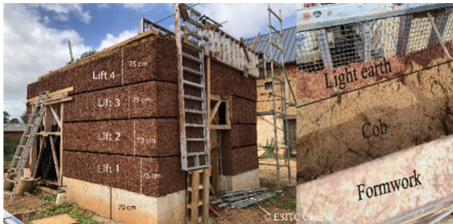
Fig. 1. View of the earthen-based building under construction in Normandy (France).
