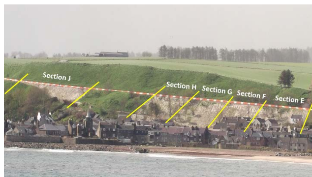
Figure 1. Site area with delineated soil nailing sections
