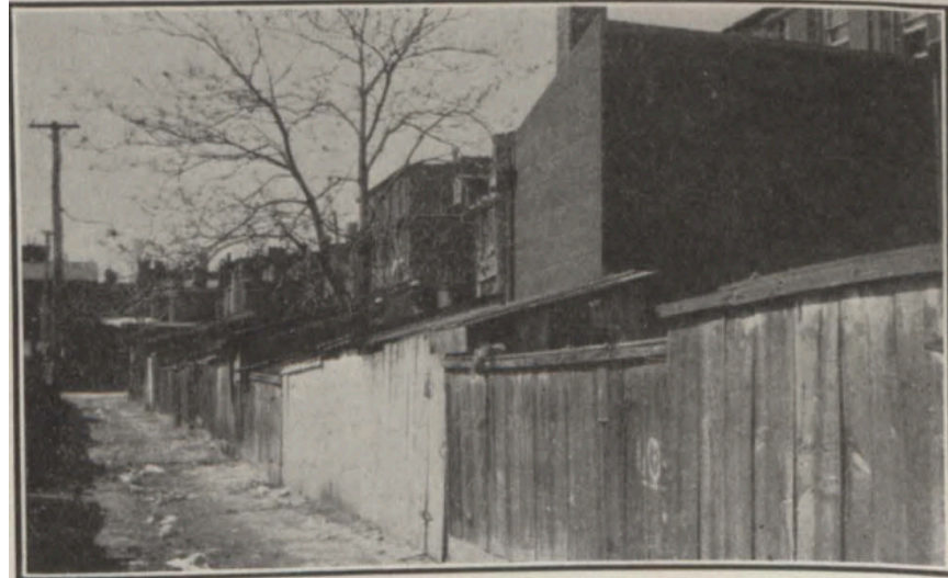
Rear of row of colored tenements. Drainage runs down through alley except when stopped and held in stagnant pools by uneven paving. Decaying fruit and vegetable matter found everywhere.
