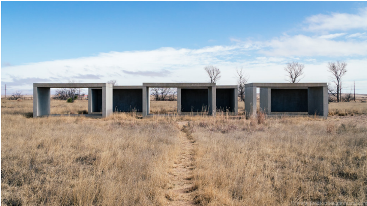
Image 18. Donald Judd, 15 untitled works in concrete , 1980-1984. Permanent collection, the Chinati Foundation, Marfa, Texas. Photo by Florian Holzherr. Donald Judd Art © 2020 Judd Foundation / Artists Rights Society (ARS), New York. 14
