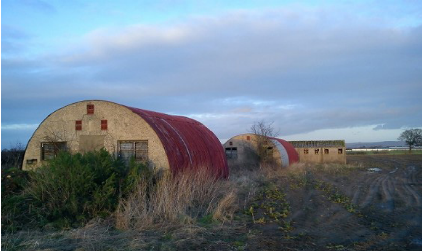
Abandoned Nissen huts at the site of RAF Skipton-on-Swale. [Image courtesy of www.lancashireatwar.co.uk ]
