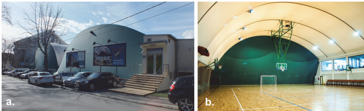
Figure 2 Double roof membrane hall: a) External view looking; b) Internal view looking
