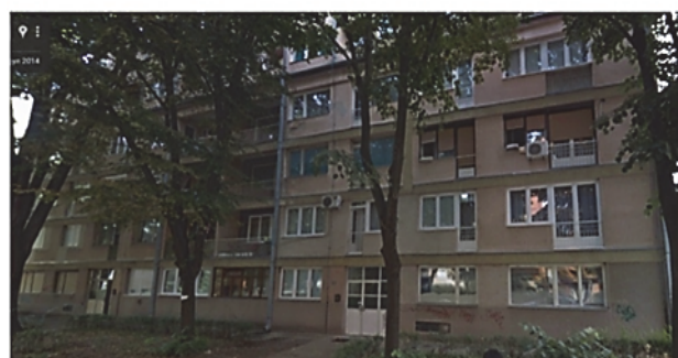
Figure 1 Observed building, "type A"
