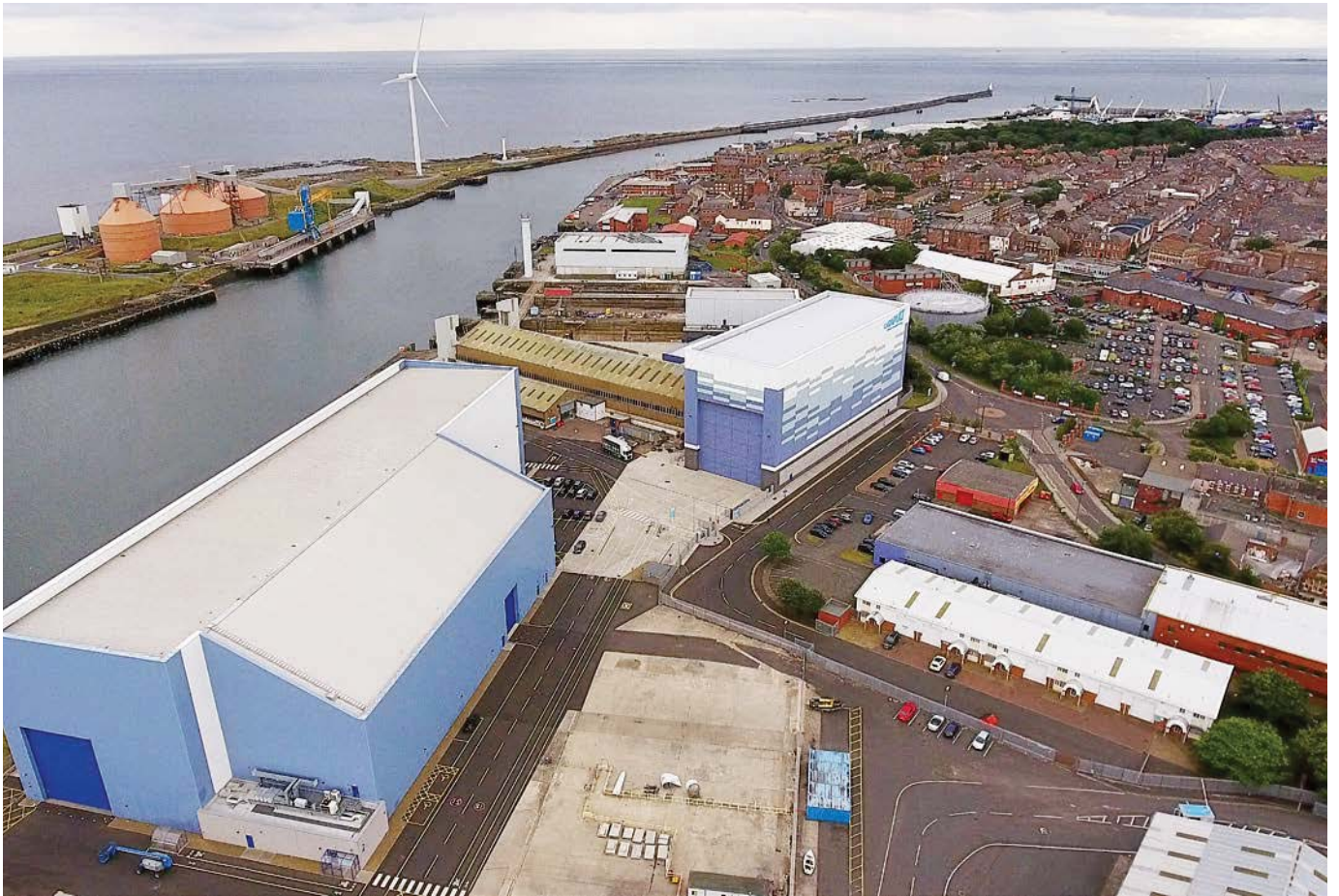
Aerial view of Offshore Renewable Energy Catapult site at Blyth, UK
