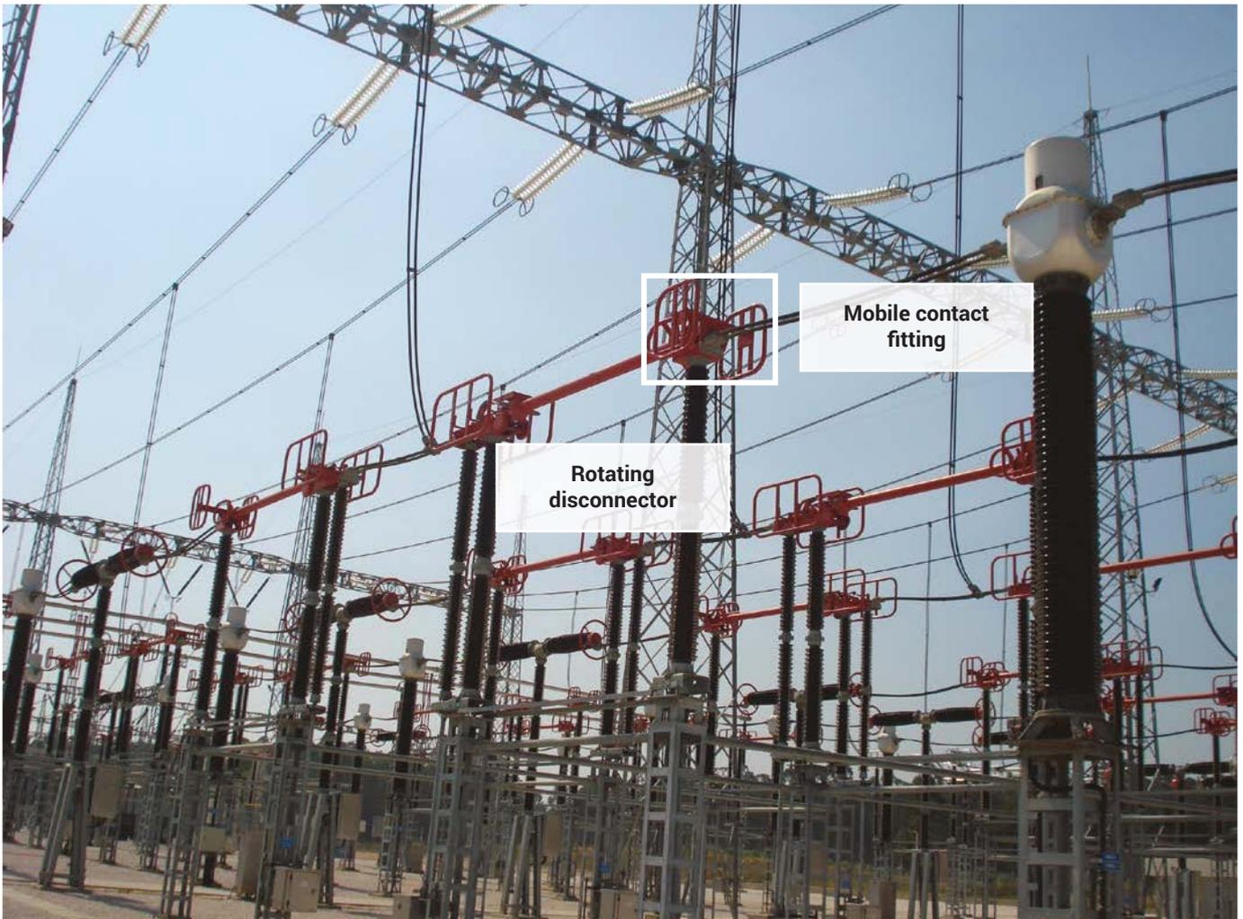
Figure 5. Rotating disconnector fitting
