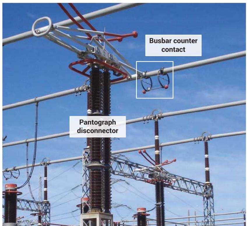
Figure 6. Pantograph disconnectors' busbar counter contact
