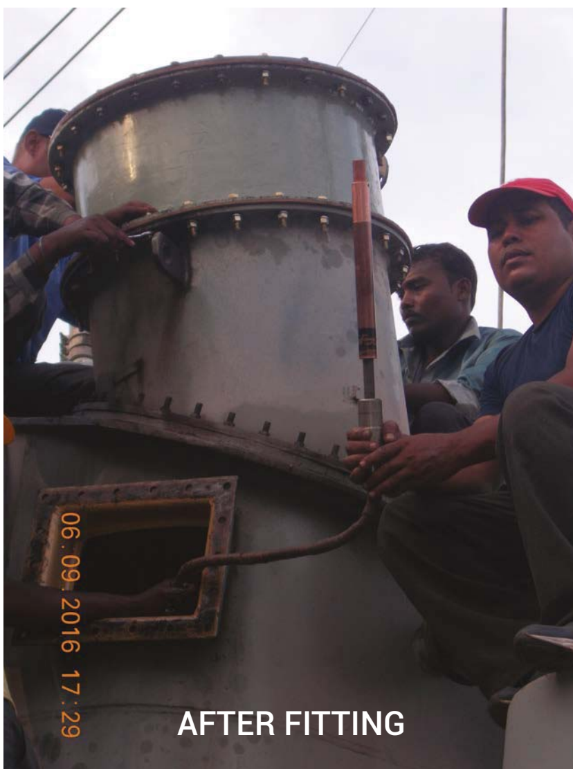
Figure 7. Fitting of extended turret adopter and extension of draw lead.
