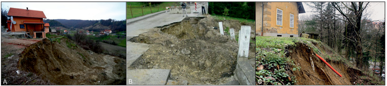
Figure 2. Examples of landslides endangering/damaging houses or public roads in the winter of 2013 in Zagreb: (A) Lazina landslide; (B) Šestinski Dol landslide; (C) Dubravkin Put landslide.
