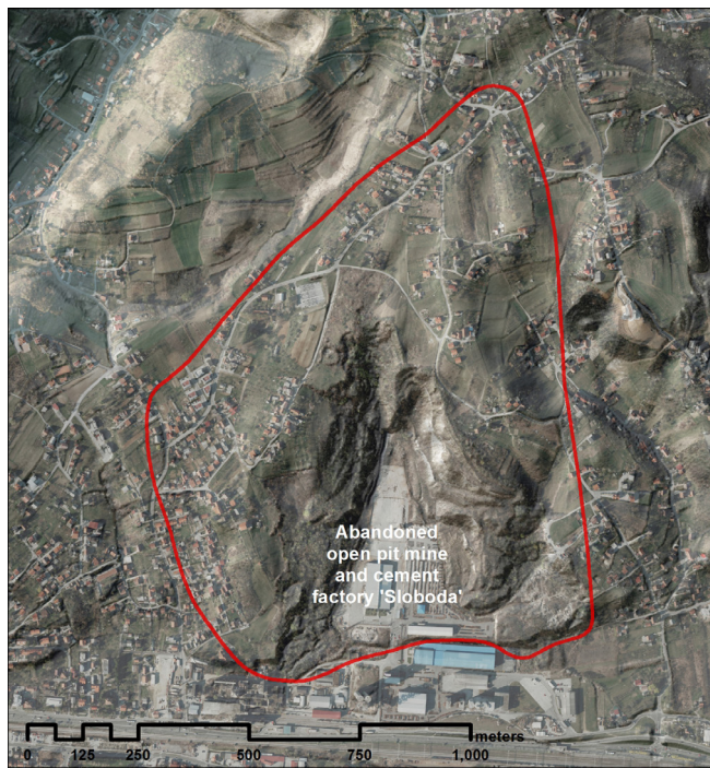
Figure 6. Kostanjek landslide area as depicted by the red line, which represents the landslide contour. In the background is an orthophoto image from March 2012. Devastated slopes of the abandoned open pit mine are expressed by rough relief forms in the middle of the Kostanjek landslide. The former cement factory 'Sloboda' was placed in the plain area in the bottom part of the landslide.
