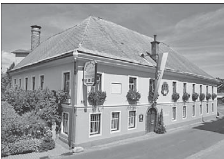
FIG. 5 "BRAEUER" GUESTHOUSE HOTEL; STCS ON THE ROOF OF THE HOTEL SL. 5. HOTEL „BRAEUER”; STS (SOLARNI TOPLINSKI SUSTAVI) NA KROVU HOTELA
