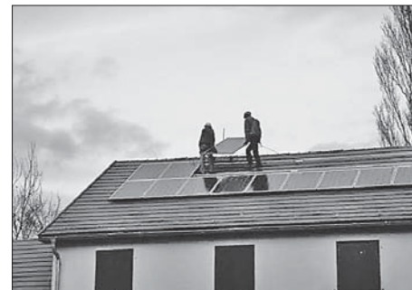
FIG. 6 STCs ON THE ROOFS OF THE LUTHERAN CONFERENCE AND MISSION HOME IN BALATONSZARZSU; PV ON THE ROOF SL. 6. STS NA KROVOVIMA LUTERANSKOG KONFERENCIJSKOG I MISIONARSKOG DOMA U BALATONSZARZSU; FN NA KROVU
