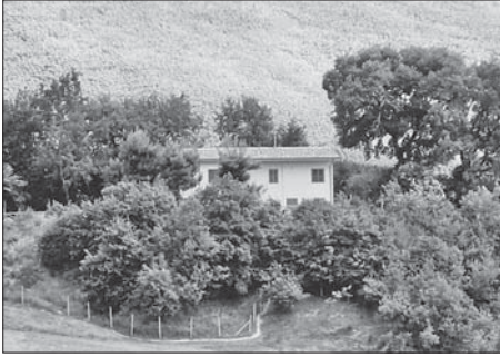
FIG. 3 THE FARMHOUSE "CASA ROSA"; PV PANELS ON THE ROOF OF THE PARKING PLOT SL. 3. SEOSKA KUĆA „CASA ROSA”; FN PANELI NA KROVU PARKIRALIŠTA
