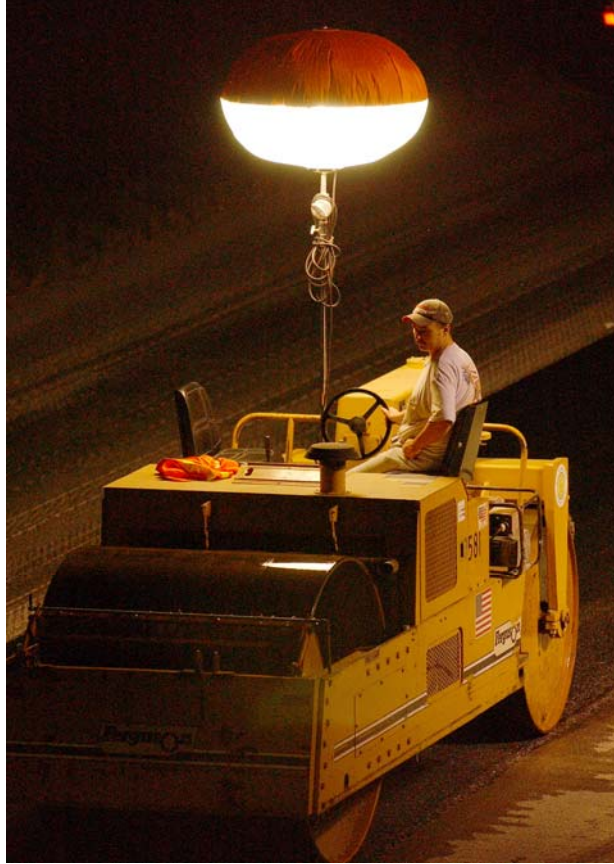
Figure 4.27. Rolling bituminous surfaces activity.
