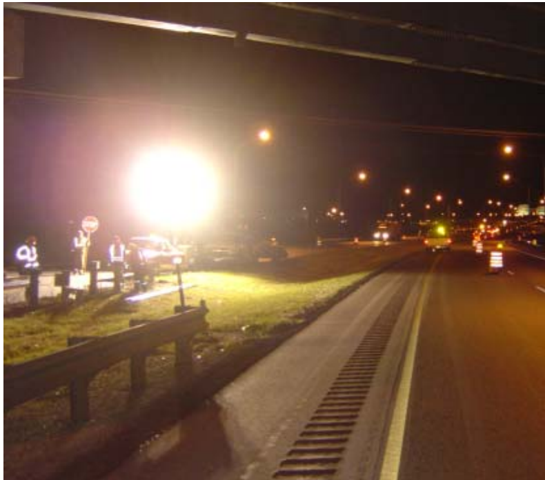
Figure 4.45. Girders repair activity.
