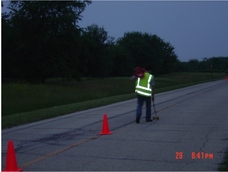
Figure 4.24. Positioning the construction cones.
