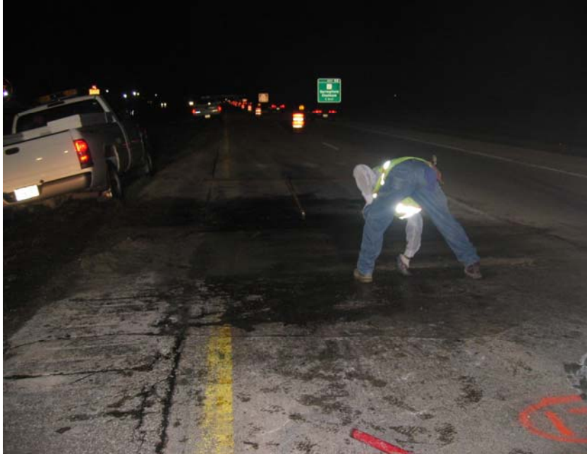
Figure 4.46. Pavement patching and repairs activity.
