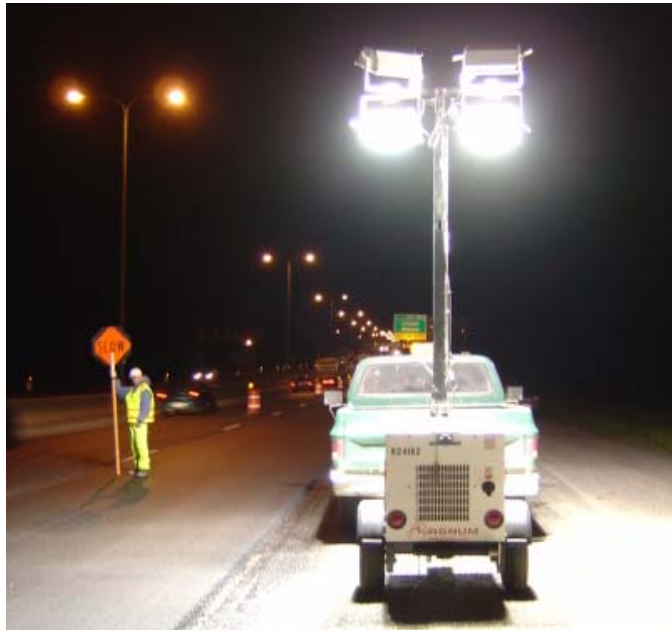
Figure 4.47. Work zone flagger station.
