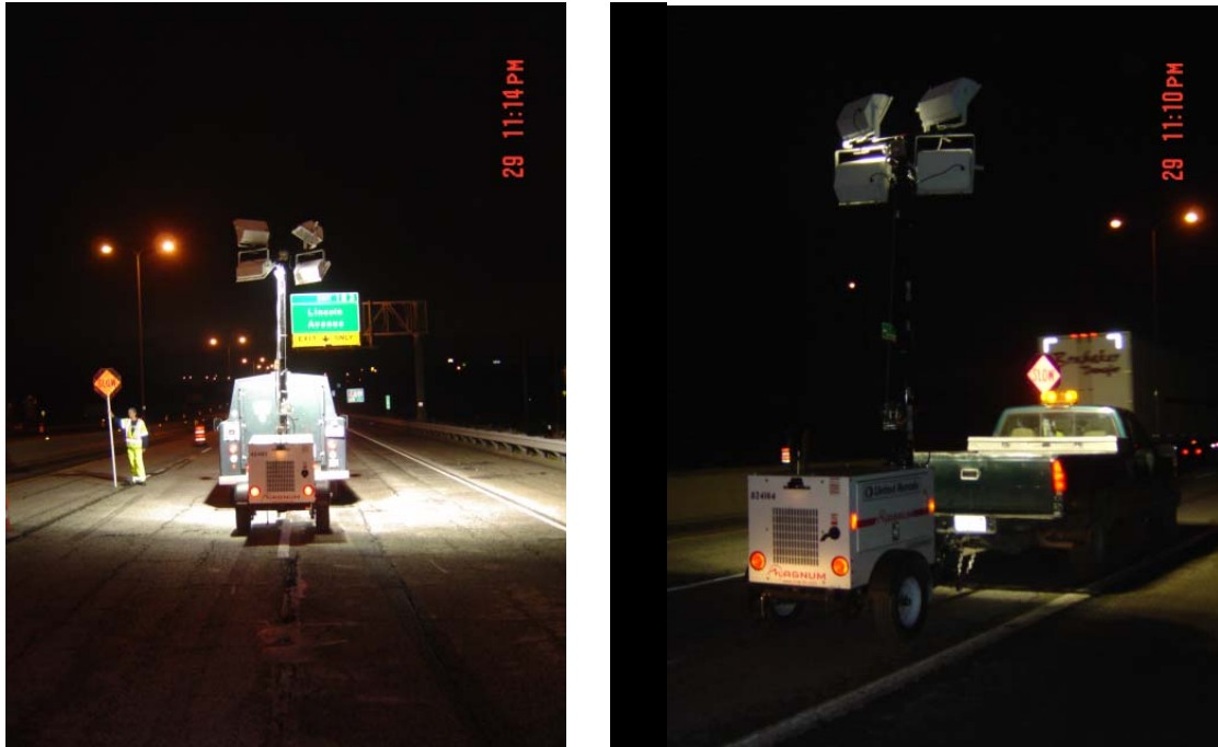
Figure 3.20. Light tower to illuminate flagger station (I-74).
