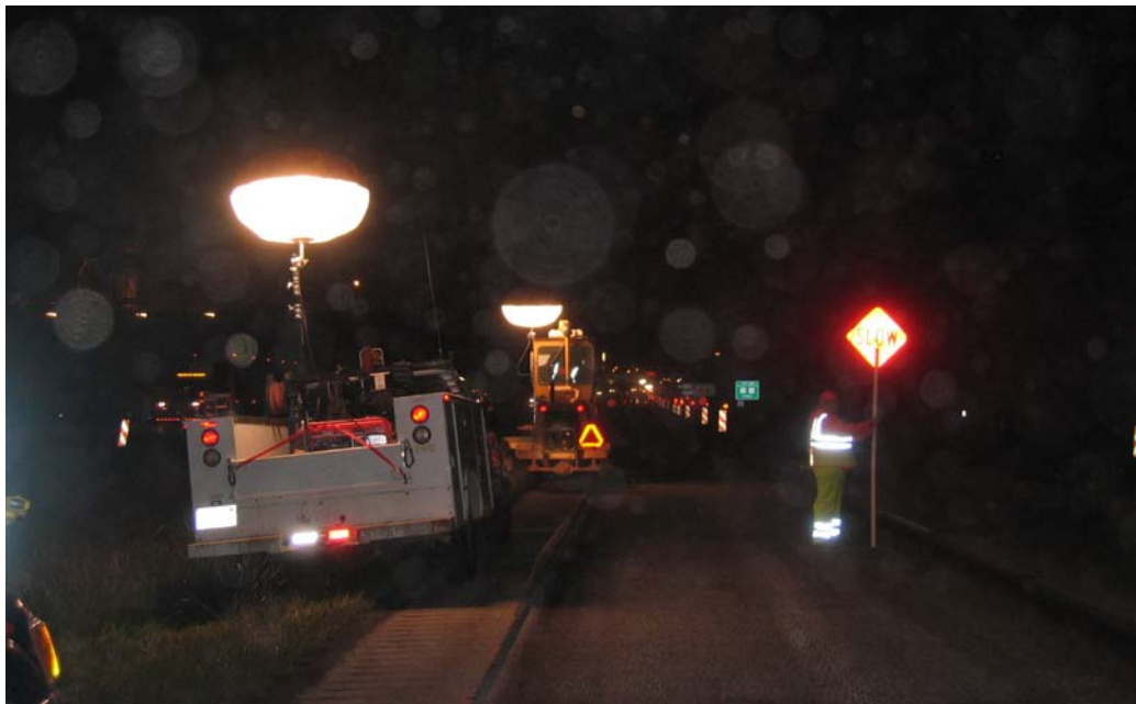
Figure 4.29. Work zone flagger station.
