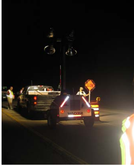
Figure 3.12. Light tower to illuminate flagger station (I-72).
