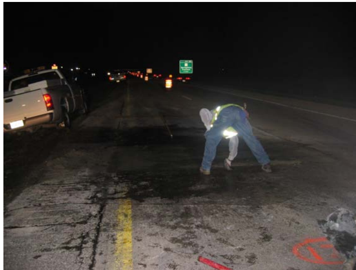
Figure 3.11. Patching operations (I-72).
