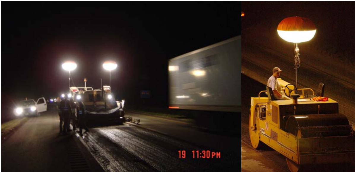
Figure 4.40. Utilization of three balloon lights in nighttime work zone.
