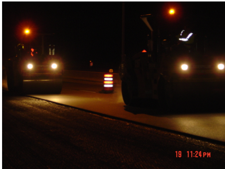
Figure 3.19. Headlights for roller (I-74).
