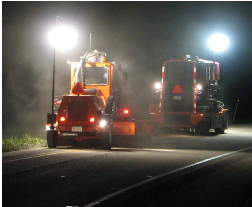
Figure 4.64. Pavement cleaning and sweeping activity.
