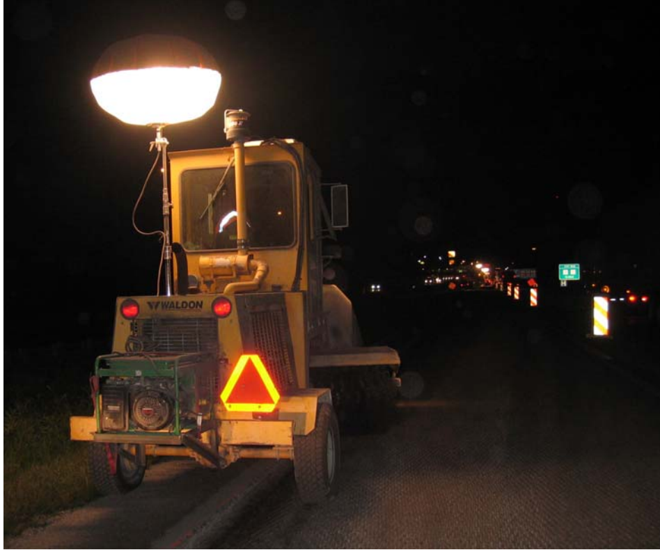
Figure 4.28. Pavement cleaning and sweeping activity.
