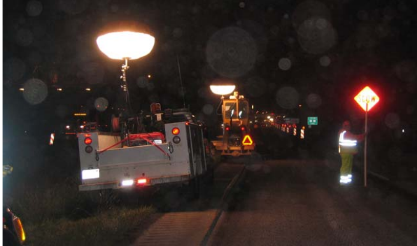
Figure 3.15. Balloon light to illuminate flagger (I-70).
