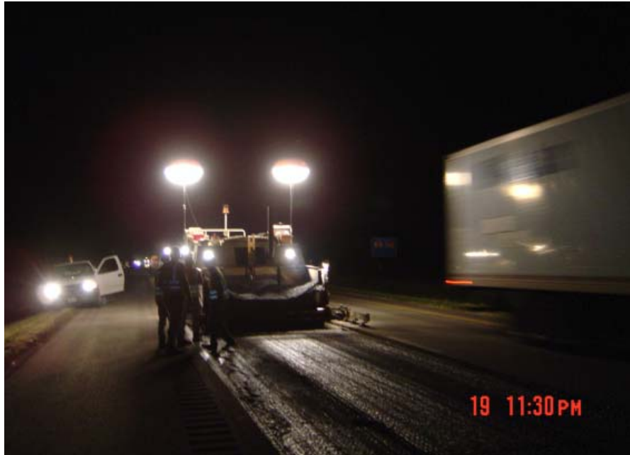
Figure 4.35. Pavement equipment using two balloon lights.
