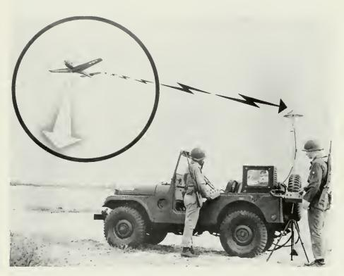
Figure 1. Unmanned aircraft send back aerial views af distant sites, using light TV equipment developed at the Army's Signal Corps Engineering Laboratories at Fort Manmouth. The camera in the L-17 drone (shown in telescopic view) can point downward or farward through the plane's belly.
