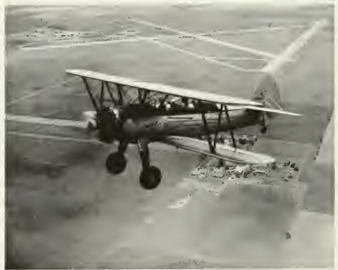
Figure 20—Conventional Biplane Showing Upper and Lower Wings and Wing Struts
