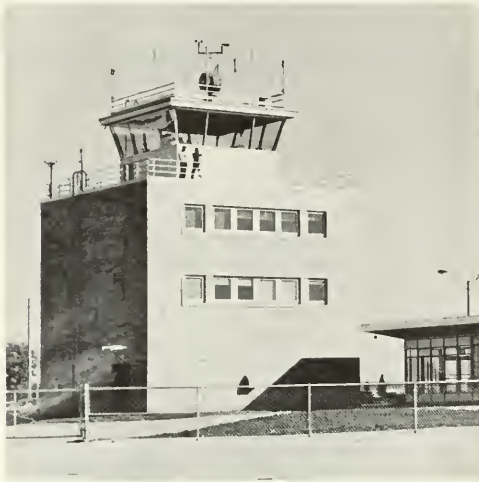
Figure 126—Airport Control Tower
