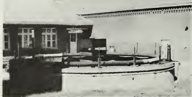
This circular concrete casing can be found just east of the Electrical Engineering Research Laboratory, and on the north bank of the Boneyard.
