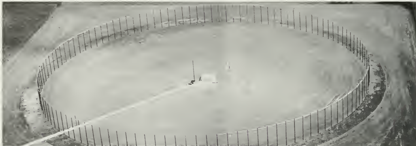
The "birdcage", a radio direction system, is located west of the Champaign campus. The system of poles is 65 feet tall and 955 feet in diameter.
