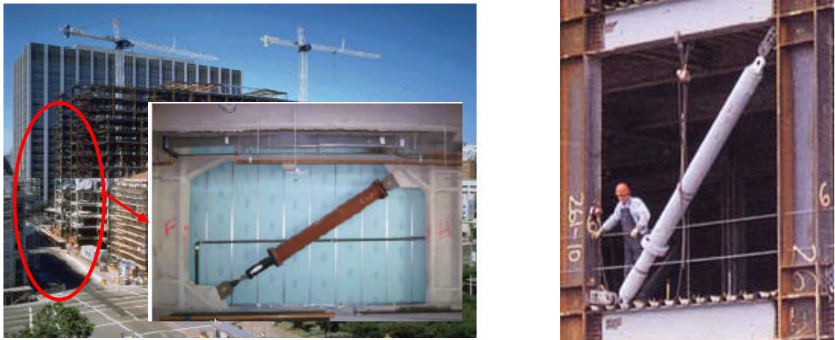
Figure 2.52. - Viscous dampers in steel framed building.
