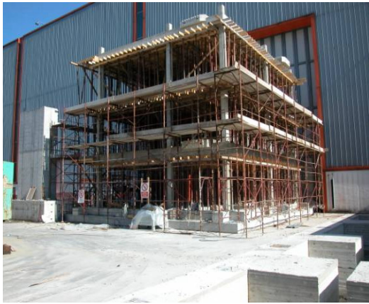
(a) Construction of the test structure
