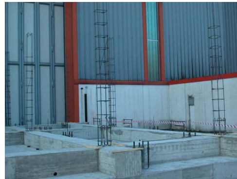
Figure 7.10 Lap splices at bottom of columns
