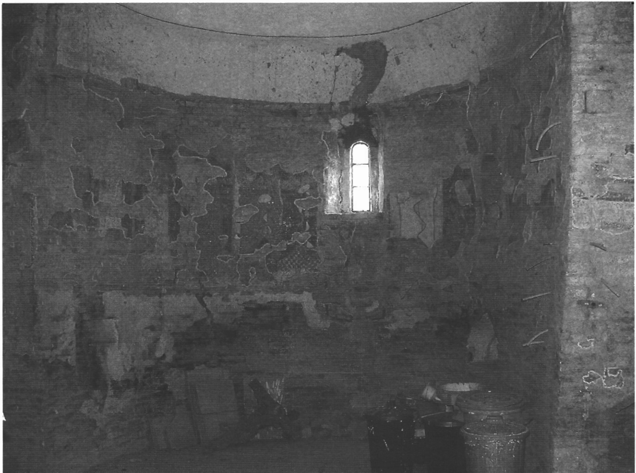
fig. 13 - Lovčić, view of the interior of the apse
