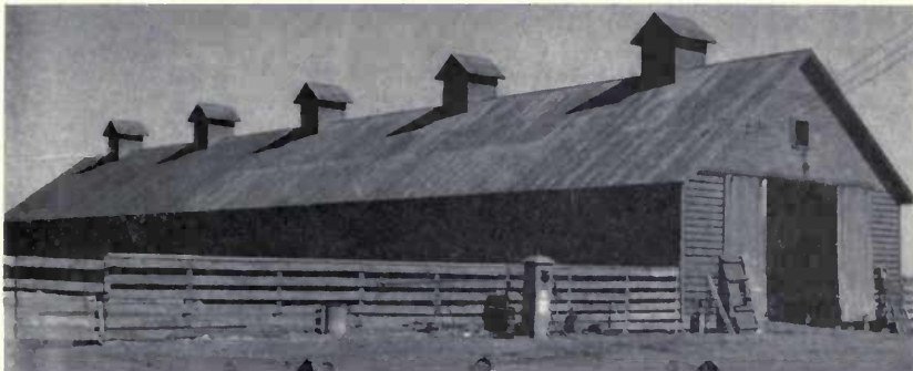
North side of crib before painting. The one-third of the roof at the left (Panels 46 through 81) was 100 percent rusty. (Fig. 2)
