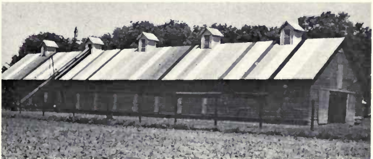
COVER PHOTO — the 150-foot corn crib on which the paint study was conducted (south side after application of first coat of paint).
