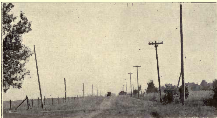
FIG. 2.—THE EXPERIMENTAL LINE, SHOWING CONSTRUCTION AT A CORNER
