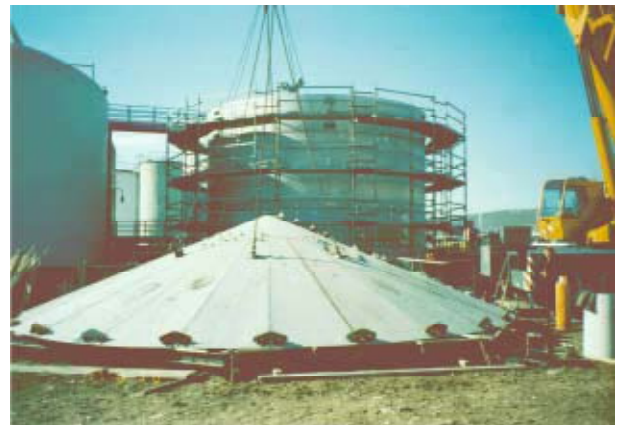
Figure 10. The storage tank's roof Slika 10. Krov rezervoara
