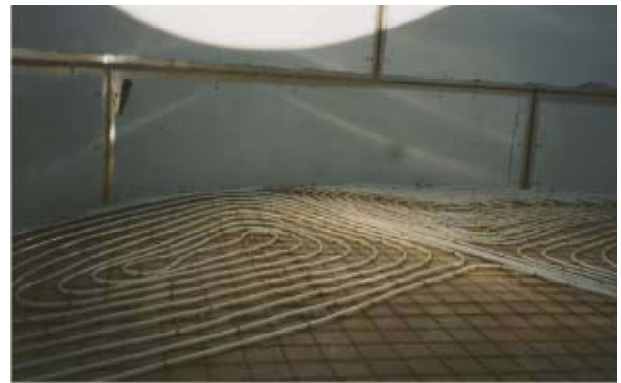
Figure 9. Heating coil on the bottom of the tank Slika 9. Sustav zagrijavanja dna rezervoara
