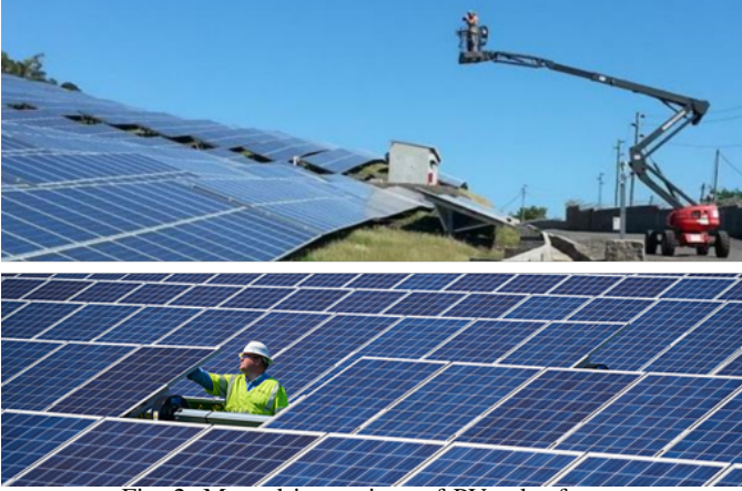
Fig. 2: Manual inspections of PV solar farms.
