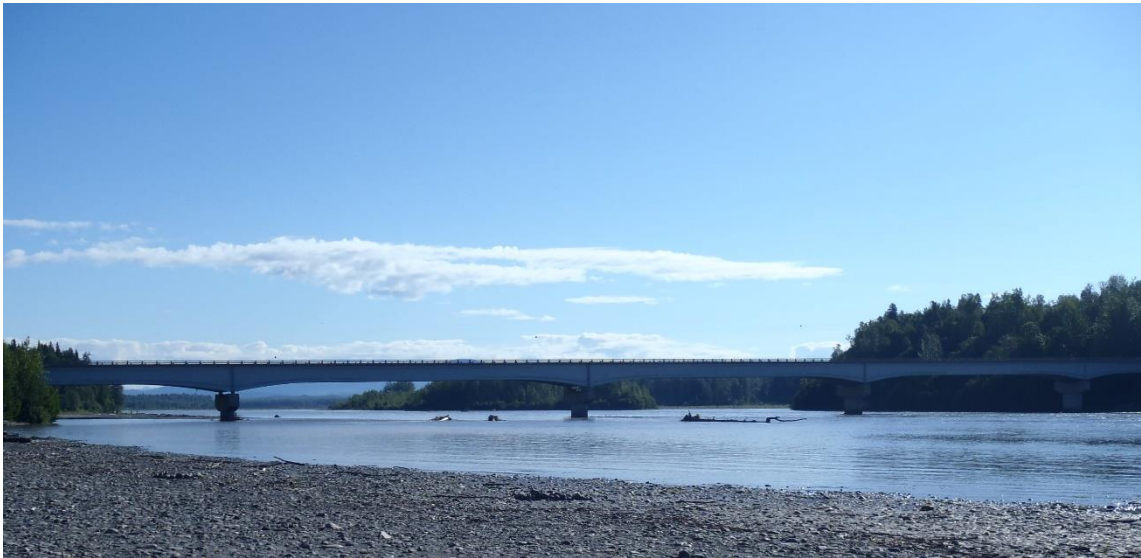
Figure 3.5. Susitna River Bridge (Alaska DOT, 2016)
