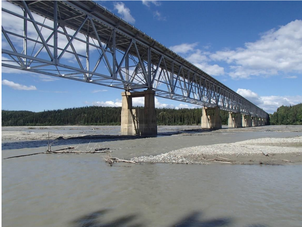
Figure 3.1. Robertson River Bridge (Alaska DOT, 2018)
