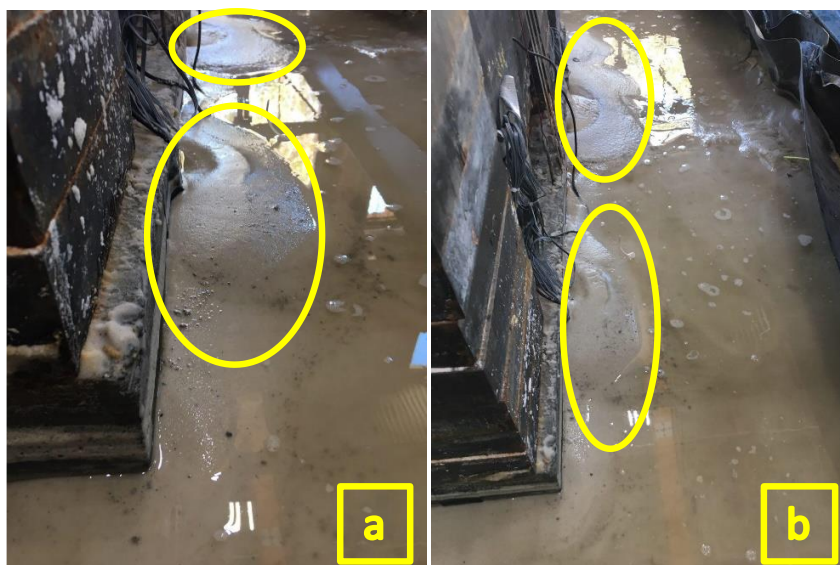
Figure 3.16. Observed sand ejecta in both (a) eastern and (b) western side of the soil box in the Helical Pile test after Shake 1.
