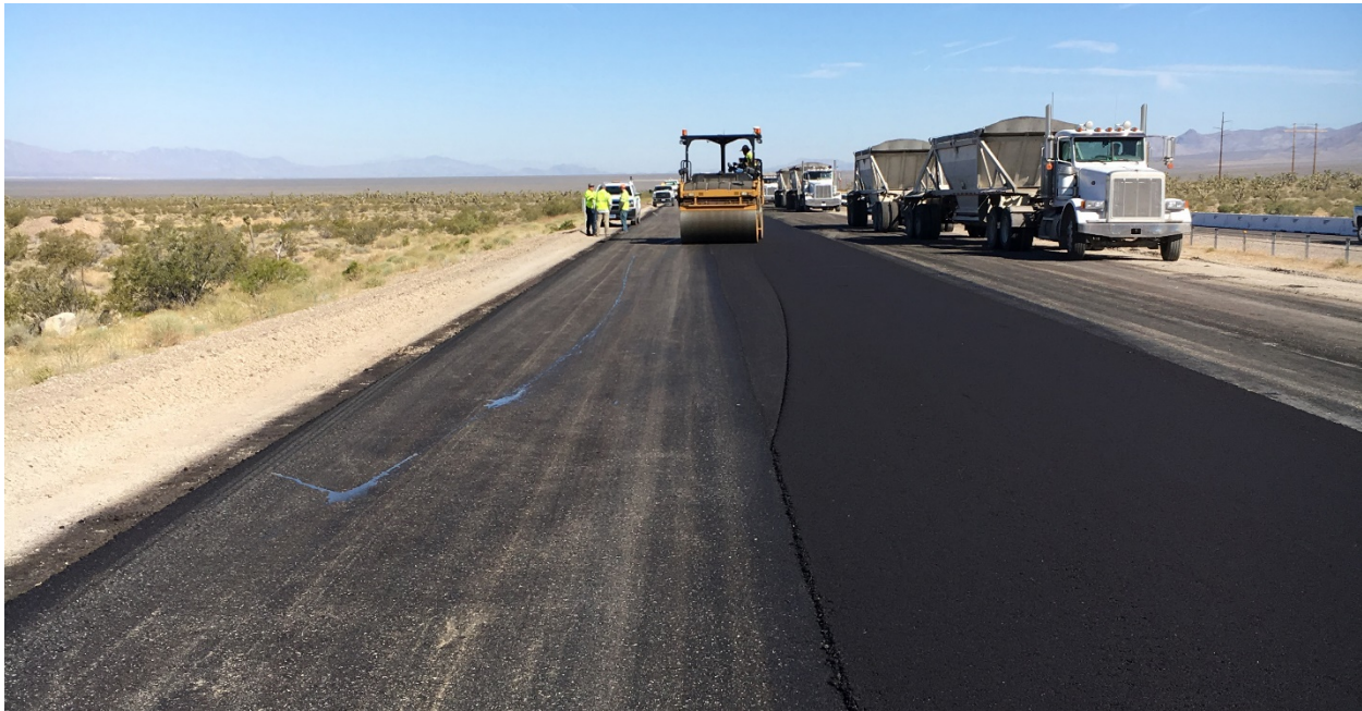
Figure 9. Longitudinal Joint Compaction
