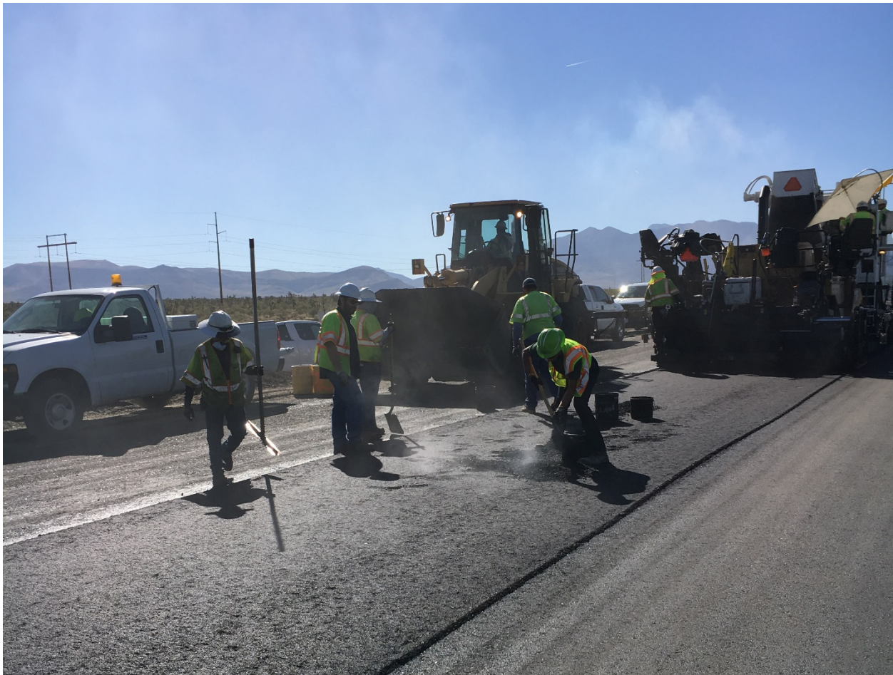
Figure 10. NDOT and Contractor Staff Obtaining Plantmix Samples from the Mat
