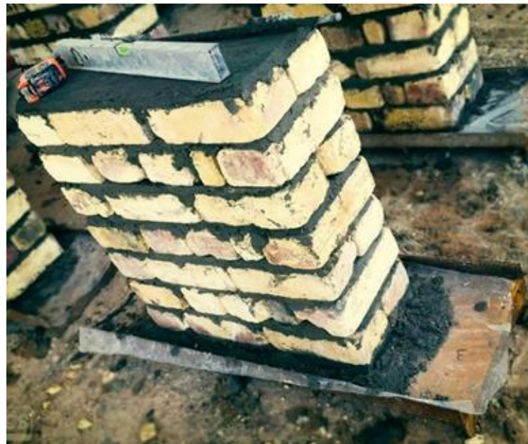
Figure 3. Finalizing the top surface of the wallettes and using underneath steel plate for lifting.
