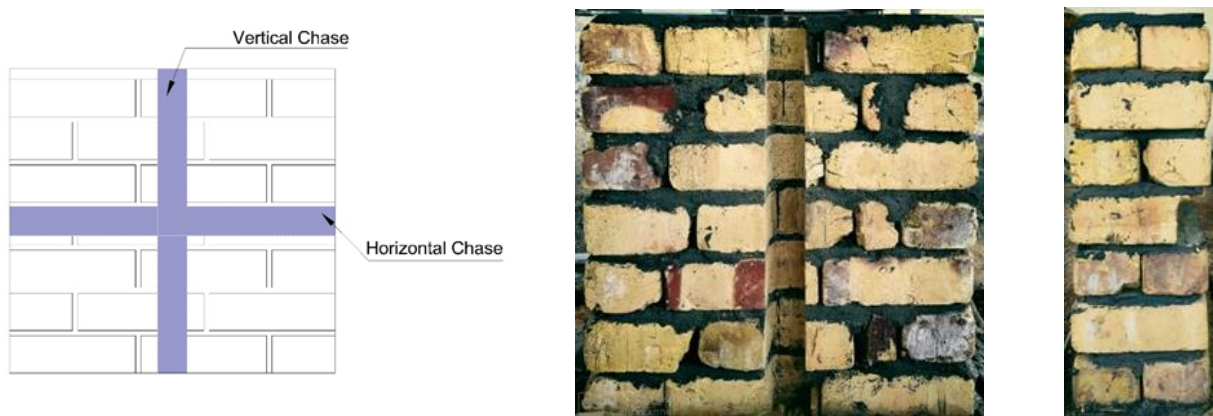
Figure 4. Creation of the vertical and horizontal chases.
