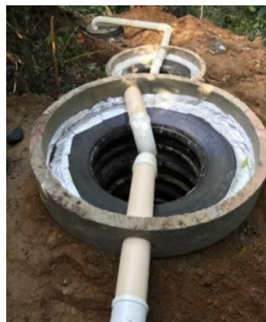
Figure 4. Tanks prepared to receive the lid. Source: Personal collection.
