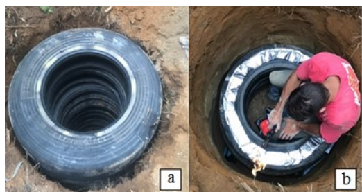
Figure 2. Overlapping tires (a), application of a bituminous layer (b).
