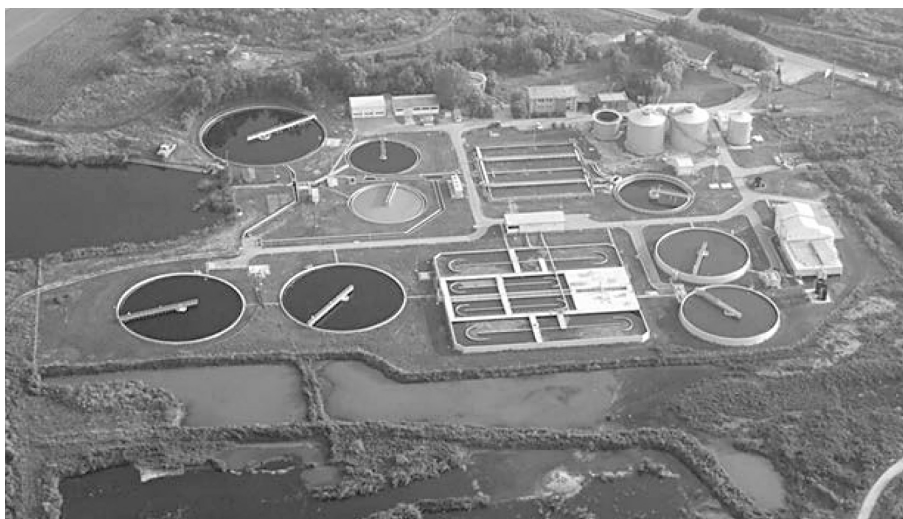
Figure 1. Wastewater treatment plant (source, http://www.vodovodsu.rs/14-Preciscavanje-otpadnih-voda )
