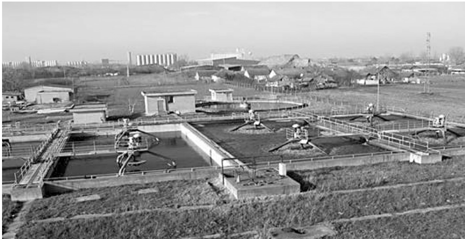
Figure 4. Pool for nitrification and denitrification (source, http://www.vodovodsu.rs/14-Preciscavanje-otpadnih-voda )
