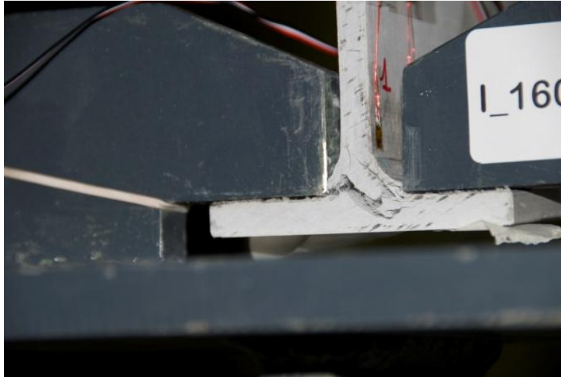
Figure 3.8. Web/Flange Junction Failure of I_160_EP_2 specimen.
