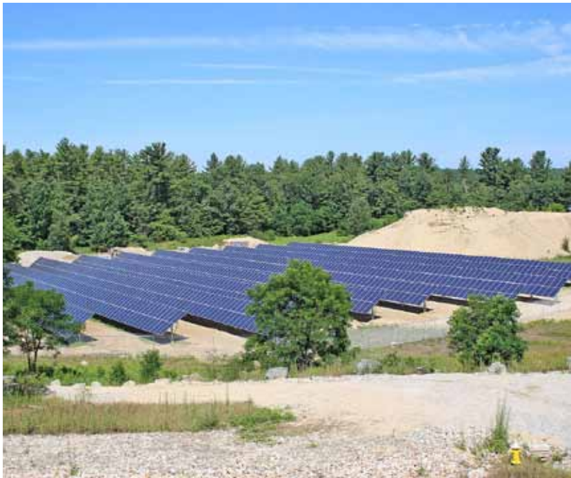
On July 21, 2016, A public ribbon cutting and tour was held at the site of the second largest solar array in New Hampshire (above) located in Lee, NH at the Packers Falls gravel pit owned by the Town of Durham. The 651-kilowatt Oyster River Forest Solar Array is the largest project to date for the installer, New England-based ReVision Energy. IGS Solar, a turn-key commercial and residential solar provider, financed and owns the array. Photo Courtesy DCAT Studios
