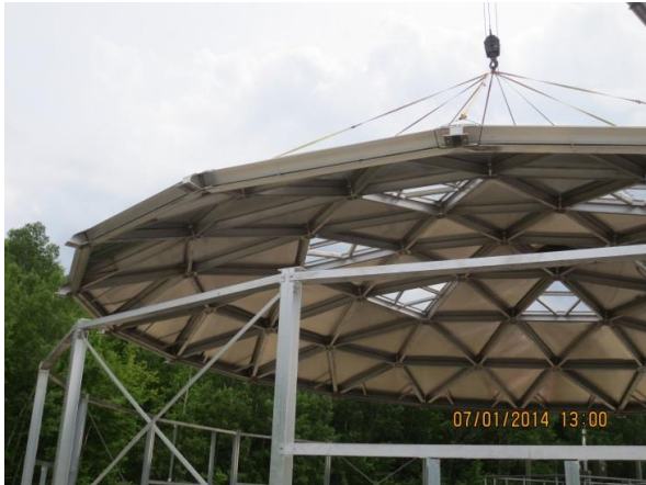
Secondary1 Dome Cover coming into place
